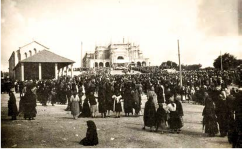
Basilica in Fatima under construction
